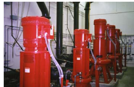
Central Contra Costa Sanitary District SCADA System
