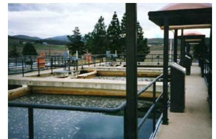
Alameda County, CA Zone 7 SCADA
